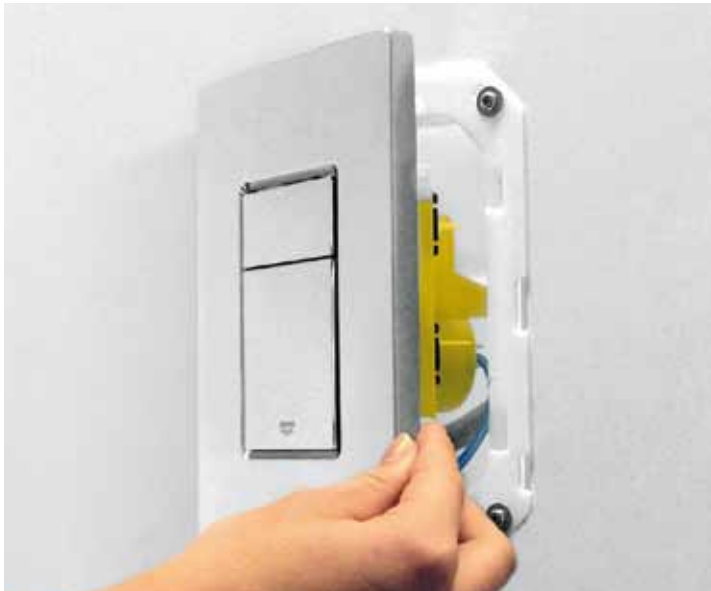
1. Open actuation of the cistern with a fingertip
